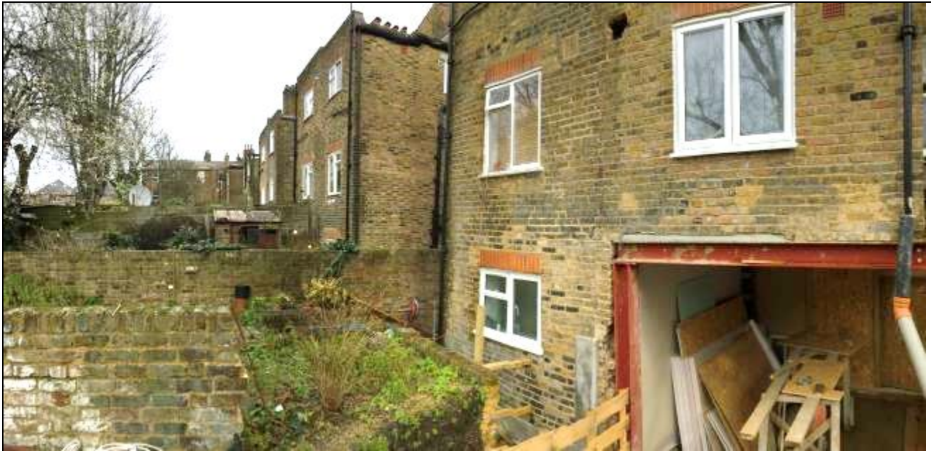
View North and boundary with No 62
